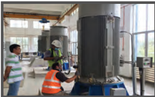
Development of tune mass damper for vibration reduction in vertical motor pump system
